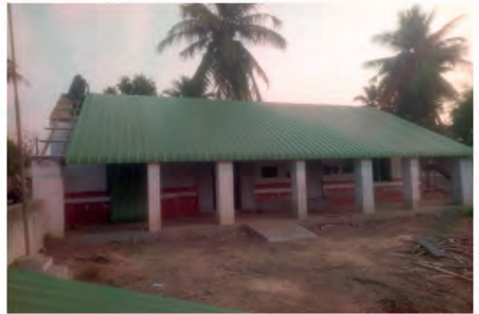
After Project completion:
