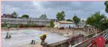
New plant within existing Unit 6
