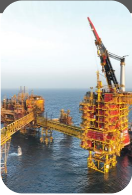
New Water Injection
