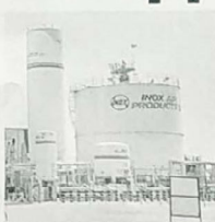
The sector has capacity to provide 3,000 tonnes of oxygen per day
