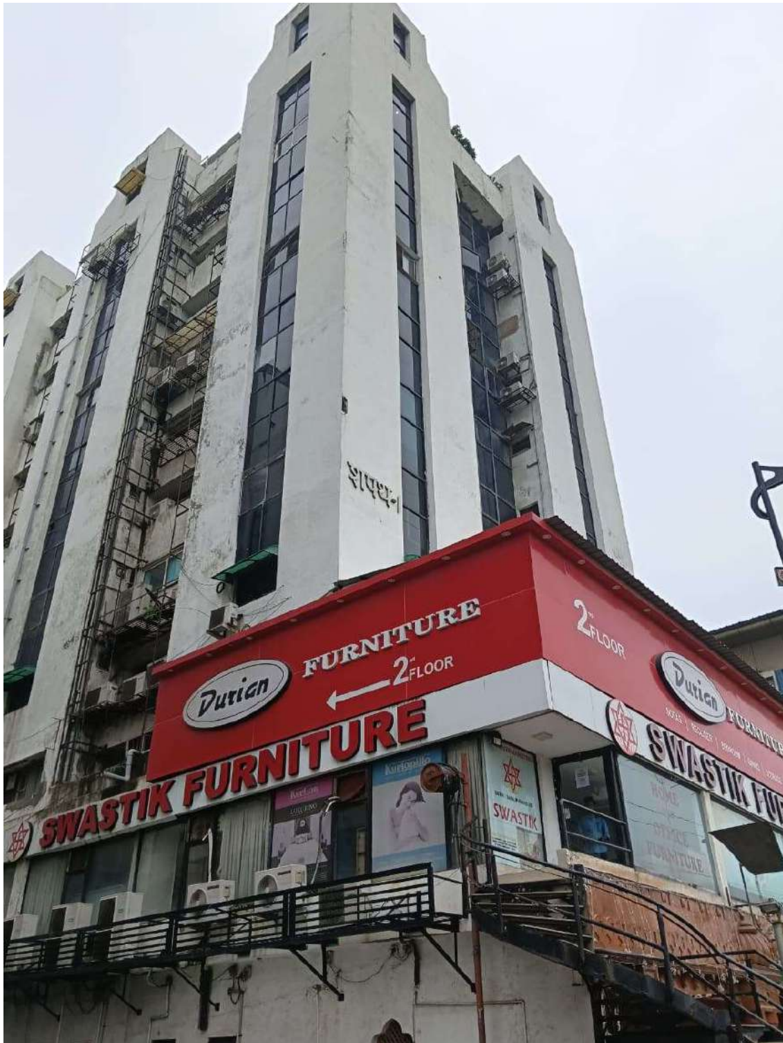
Photograph 1: Exterior view of Shapath-1 / Shapath Complex, wherein the Registered Office of the Corporate Debtor is situated.
