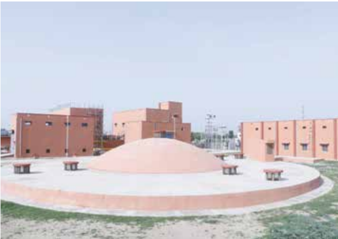
3000 KL Clear water REservoir, Jawai, Rajasthan India
