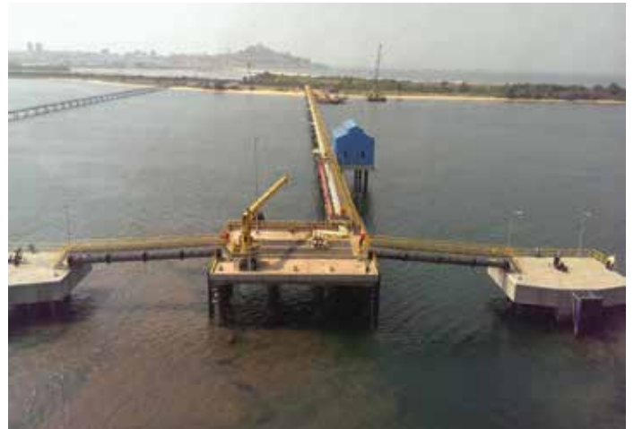
Fuel Unloading Facility at Free Port of Monrovia, Liberia
