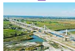
Assam-Meghalaya Bridge Corridor India's Longest Extra-Dosed Bridge Video: Explaining Pier Table
