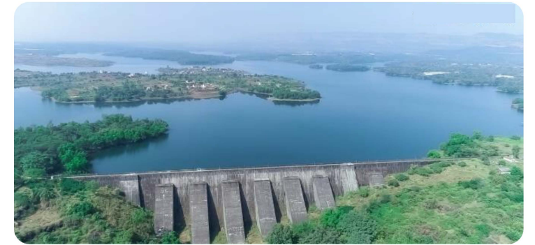
348 MCM Thokarwadi dam , Bhivpuri
