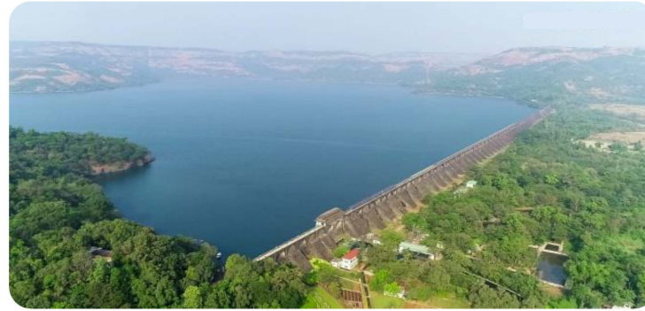
72 MCM Walwhan dam , Raigad
