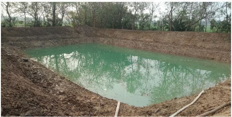
Pond excavation for water harvesting
