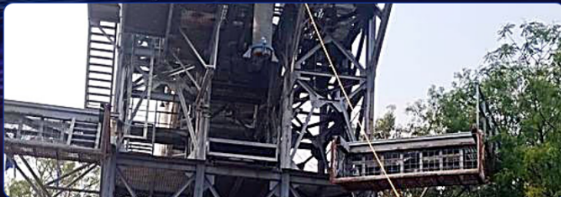
1,000 T CRM horizontal structural test facility
