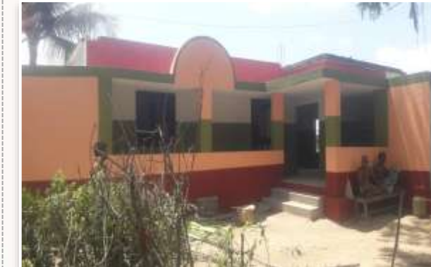
Reconstructed Pre-primary Education Centre at Bamonara Village, East Medinipur
