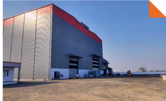
Thermotech Systems Limited (149.60 kWp)
