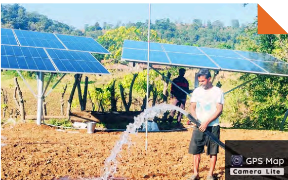
DGVCL (2760 Nos. Solar Water Pump)
