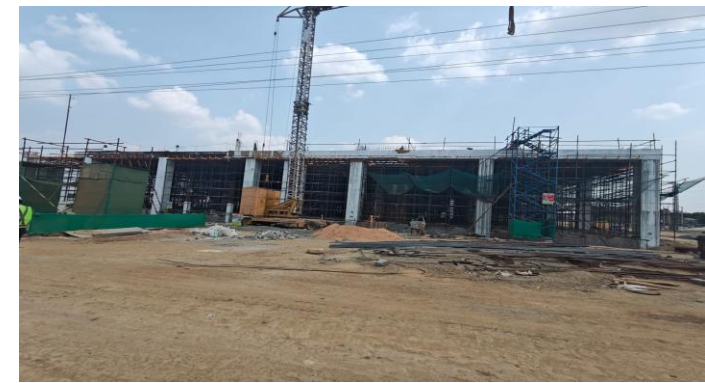
Foundation and structural work underway
