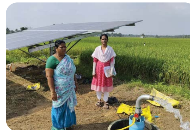
10 HP DC Submersible Water Pump at Tiruvapur, Tamil Nadu
