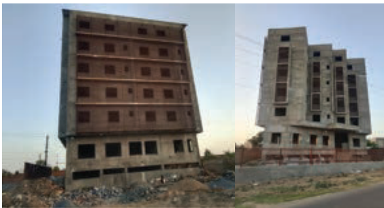
Ongoing Construction of an Educational Building
