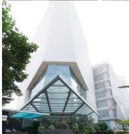
CCIL Bhavan Phase I Upto 6 th floor
