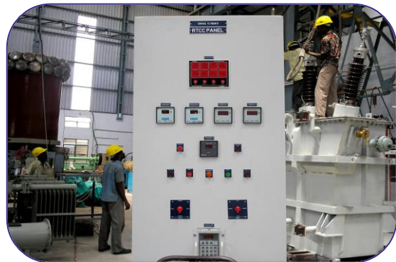
RTCC Panel Assembly
