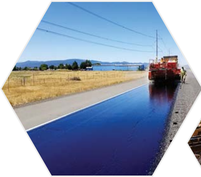
Road Construction Blue Coating Technology
