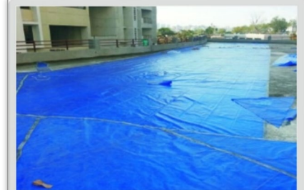
CIVIL ENGINEERING APPLICATIONS
