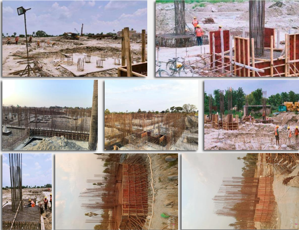
Pile Cap Work At VRM, Bihar
