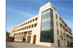
Heat Exchanger Plant
