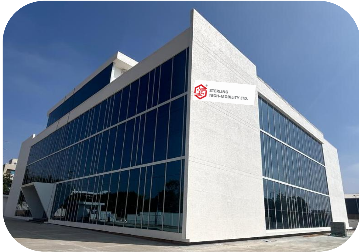
STML Manufacturing Plant- Bengaluru
