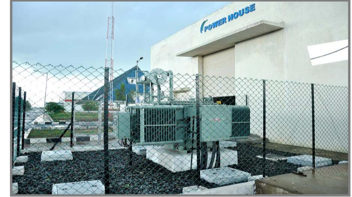
Project Name: Win Wind Energy Ltd Client: Vestas Location: Chennai Transformer Rating: 1250 KVA
