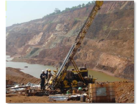
Core drilling for Chromite for Tata Steel Limited
