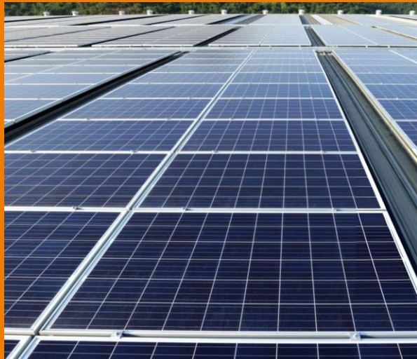
JREDA Government Building, Jharkhand
