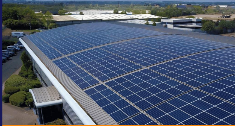
Solar Industrial Rooftop
