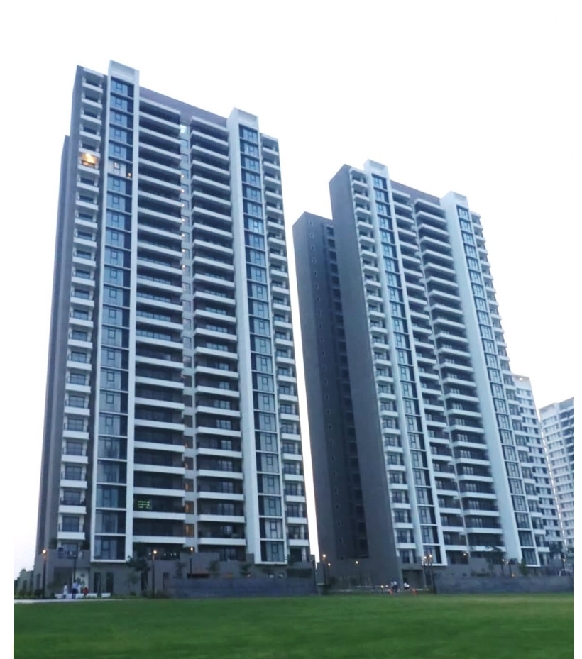
3 Towers : A2 & B2 –( S+ 18 floors) & C2 –(G+24 floors) Total SBA completed in Q3-FY23 – 457,608 sft (240 units)
