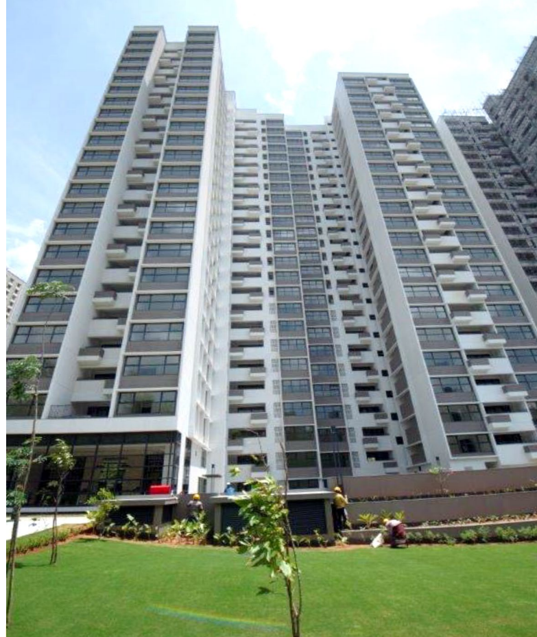
Wing 2 comprising 1 Tower of G+ 24 floors Total SBA completed in Q3-FY23 – 135,413 sft (74 units)
