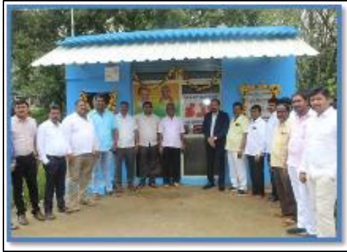
RO Water plant installed at Agara district benefitting approx. 1000 families
