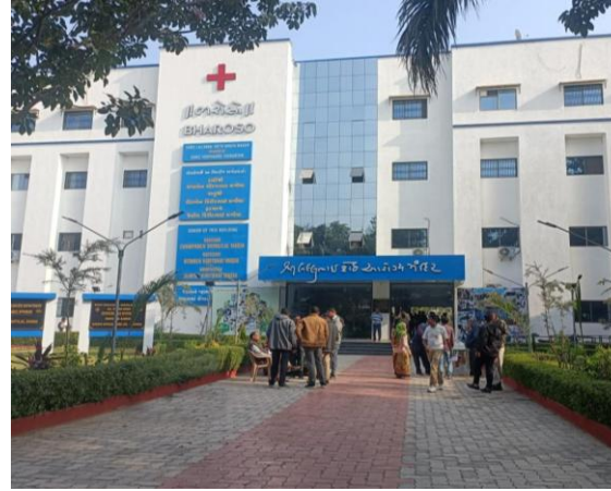
Savarkundla Hospital, Gujarat
