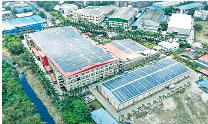
Solar Panel at our Plant
