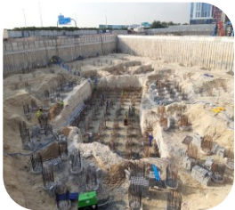
De-watering Project at Hyatt Place Hotel, Dubai
