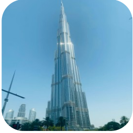
De-watering Project at Burj Khalifa, Dubai
