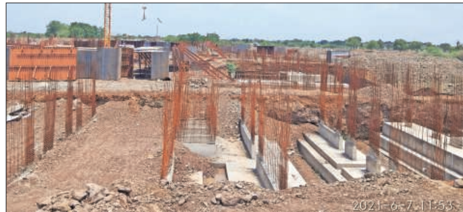
Work in progress on Light House Project in Rajkot on Monday. Gopal Kateshiya
