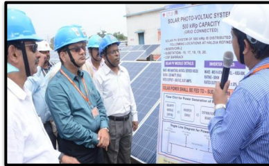
Rooftop Solar Project IOCL (Haldia & Panipat Refinery)
