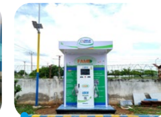
Glimpse of BPCL Project
