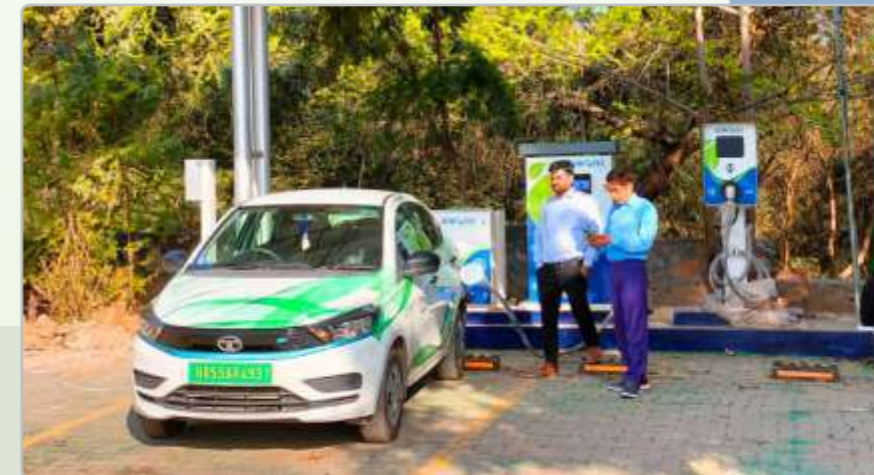
Glimpses of Solar Powered EV Charging Carport
