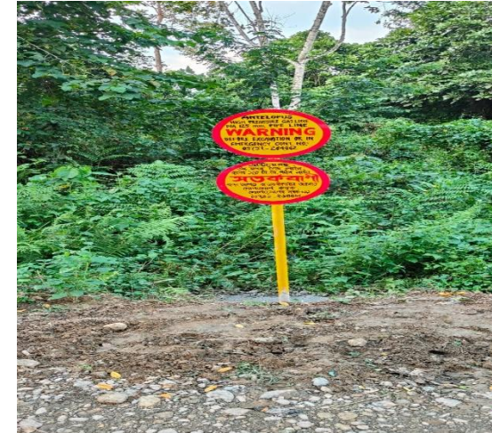
MDPE Pipeline markings
