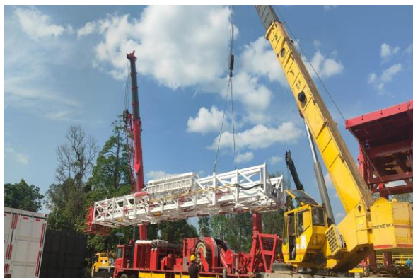
Rig building in progress
