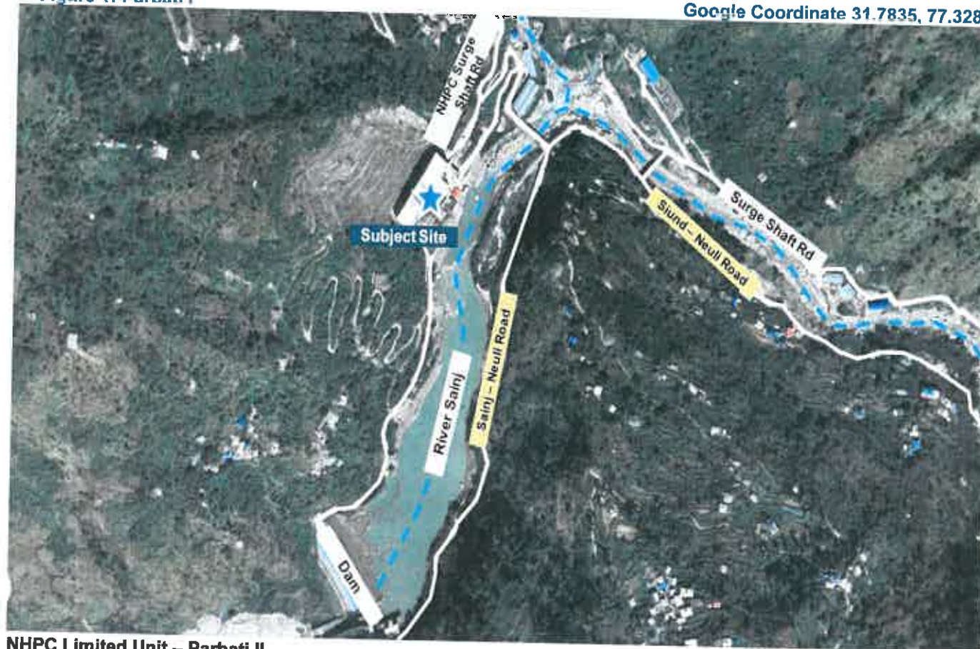
NHPC Limited Unit – Parbati II
