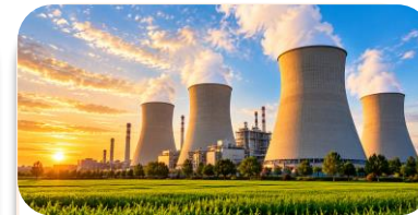
THERMAL POWER GENERATION
