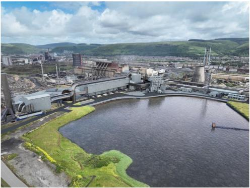
Artist's impression of the extended steelplant in Port Talbot which will house the new Electric Arc Furnace and conveyor feeding scrap steel into the furnace.
