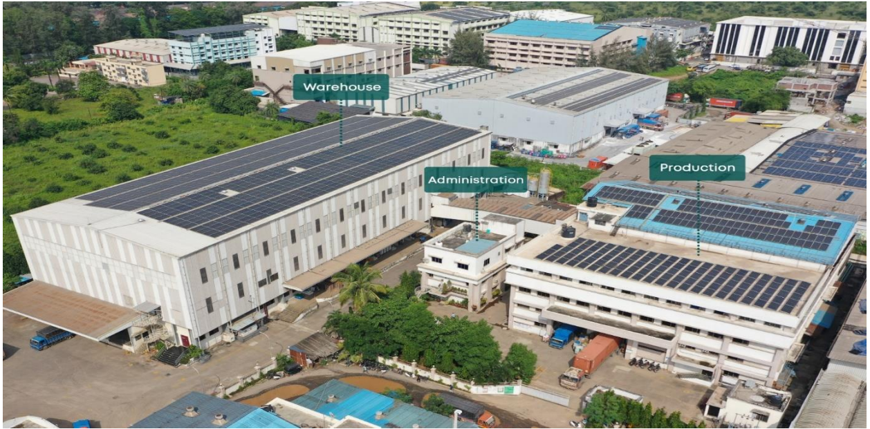
Above: photo of the Daman Facility.
