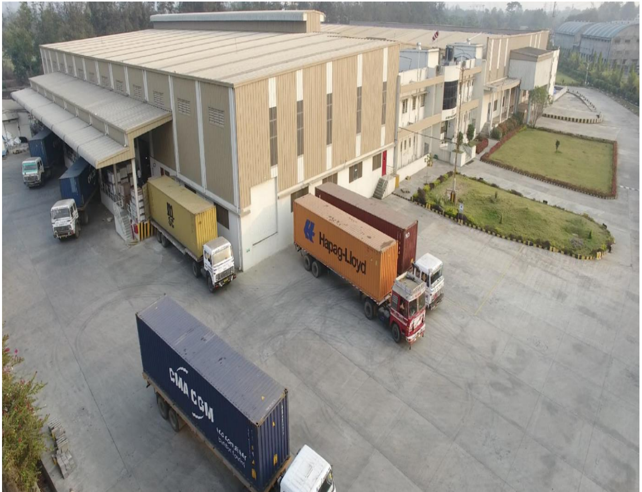
Above: photo of the Silvassa Facility.
