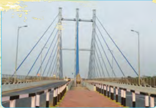
Cable Stayed Bridge, Bardhaman
