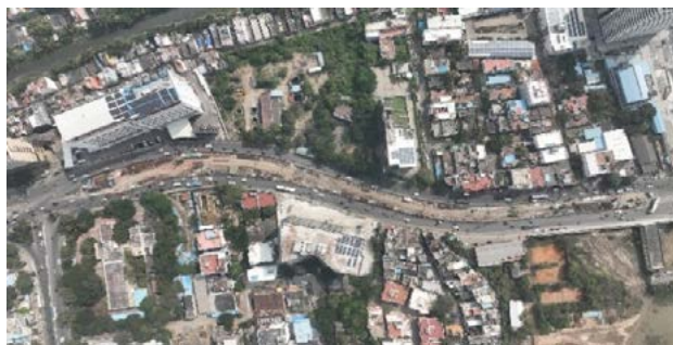
UG-05 – TARAMANI RAMP (Diaphragm wall works in progress)
