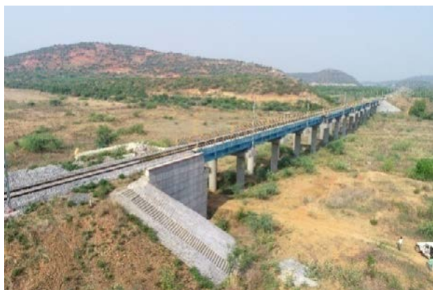
New Rail Line between Krishnapatnam &amp; Obulavaripalle
