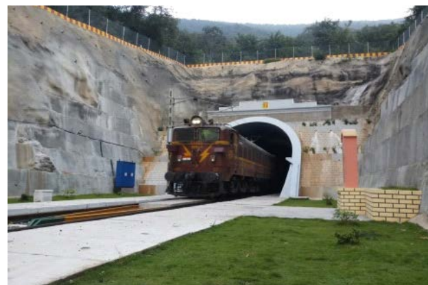
Tunnel on KRCL Line
