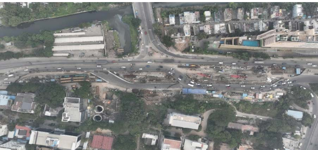
UG-05 – TARAMANI STATION (D Wall in progress – Traffic Diversion – Birds Eye View)
