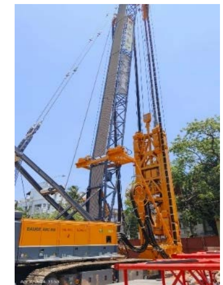
D Wall in progress with RVNL Bauer Make Trench Cutter
