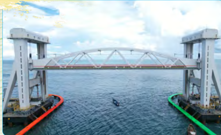
New Pamban Bridge
