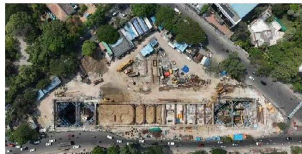
UG-04 – GREENWAYS STATION (Station Roof slab in progress – Two Pours completed)
