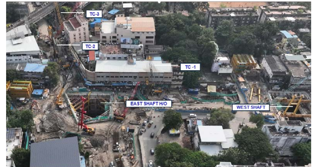
UG-04 – THIRUMAYILAI STATION (D Wall in progress with 3 Trench Cutters – East & West Shaft – Birds Eye View).
