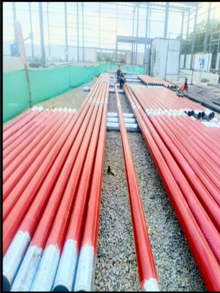
Pipe stacking , Cleaning and Painting
