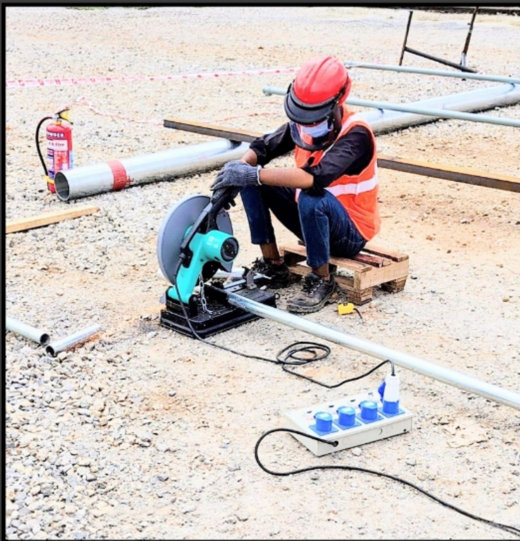
Pipe Cutting with proper PPEs and Suitable Fire extinguisher
