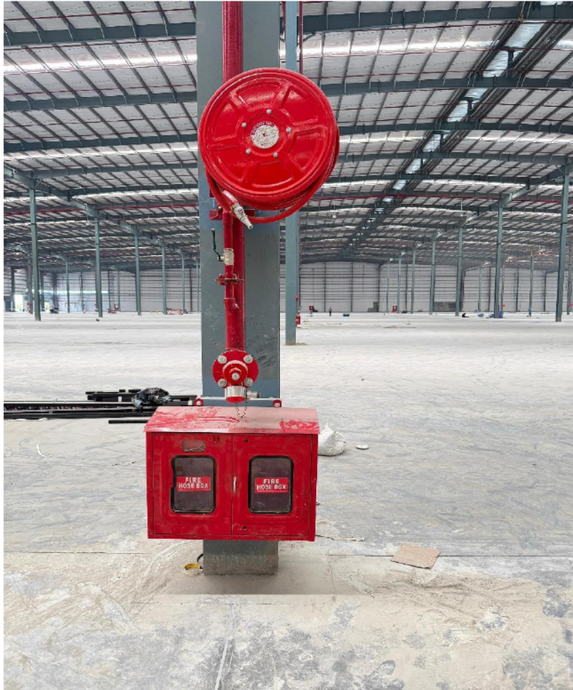
Internal Work-Hydrant Valve ,Hose Box & Hose Reel Installation
