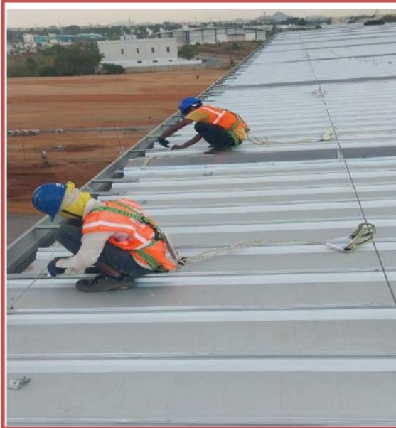
LPS WORK IS GOING ON WITH FULL PPE's ALSO WITH LIFE-LINE.
