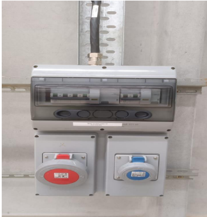
Neat installation with proper termination in the combination industrial socket
