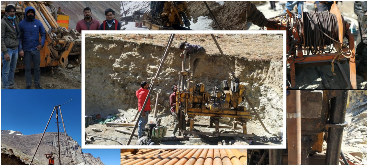
IRITES' team undertakes geotech investigation for a tunnel project in Leh
