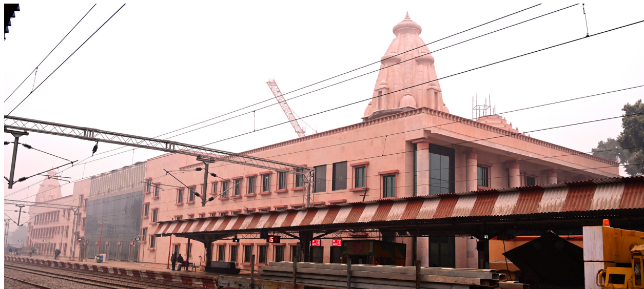
The Ayodhya Railway Station being redeveloped to offer state-of-the-art passengers amenities
