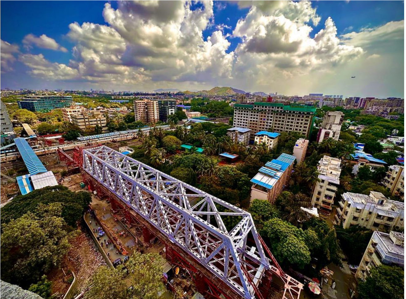
Safety & Quality Assurance services for Mumbai's longest ROB on the Central Railway Tracks at Vidyavihar Station
