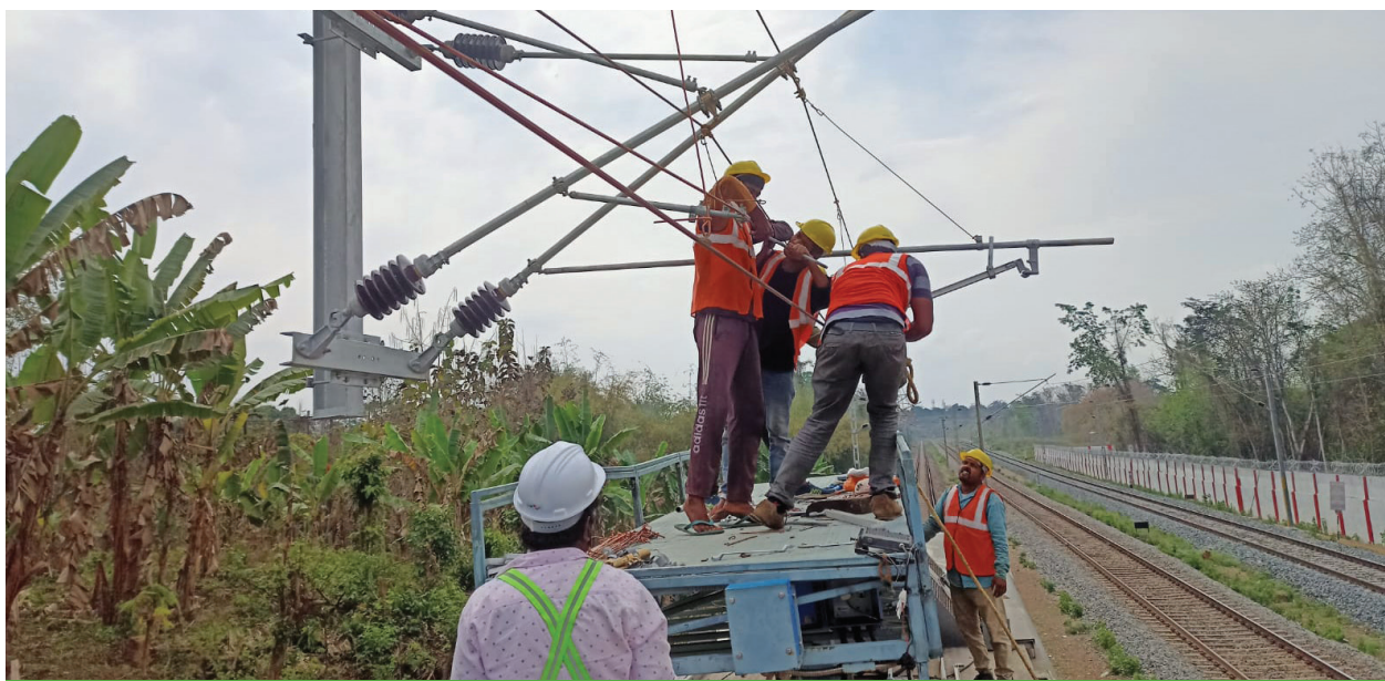
Railway electrification works underway at the Lumding-Badarpur Section
