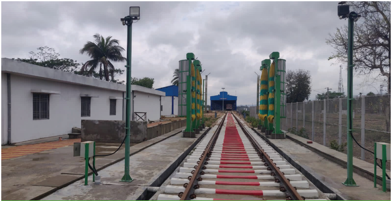
The DEMU/MEMU Shed at Lumding, Assam, a RITES project
