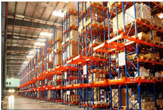
RACKING SYSTEM INSIDE ADC
