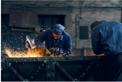
Fabrication & Erection of Structural Work on Procurement & Construction Basis
