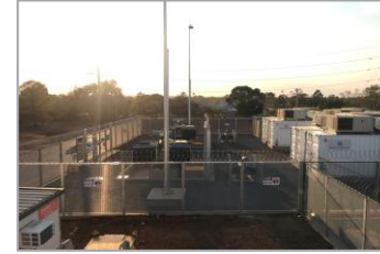
STATCOMs Upto 5 MVAR ratings
