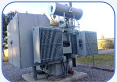
Shunt reactors
