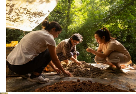
Preparing mud plaster mix using natural materials to promote eco-friendly and sustainable construction practices, West Bengal
