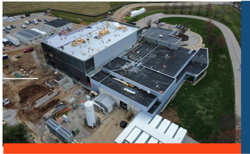
Ongoing expansion in Lexington
